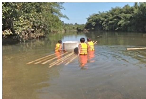
Fig. 13 – Floating a cement ring on a bamboo raft to its in-stream location for fish-raising
